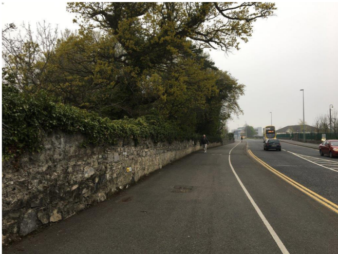
EXISTING STONE BOUNDARY WALL GREENHILLS ROAD
